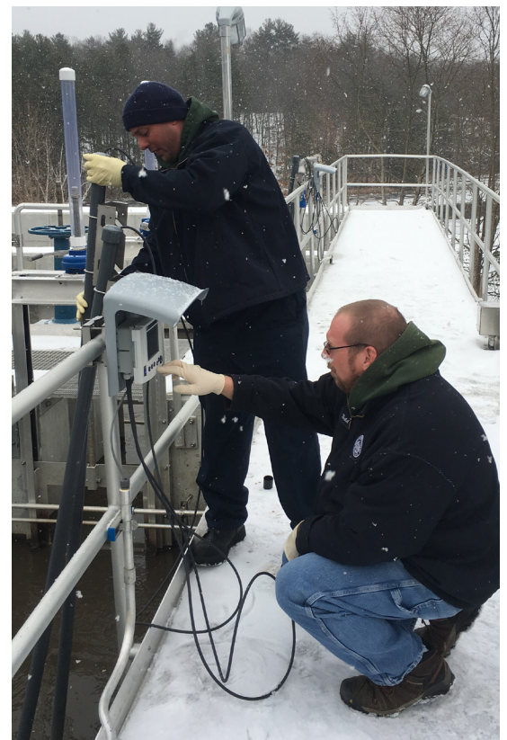
Todd Gianotti and James Barlow performing maintenance on their IQ SensorNet system at Newmarket WWTF
